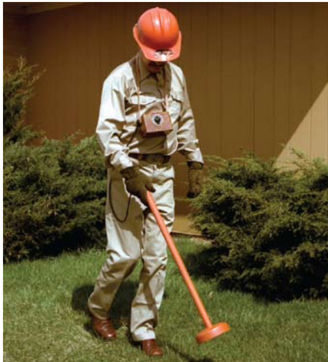
Locating the buried cable (Cat. No. T4030572)
